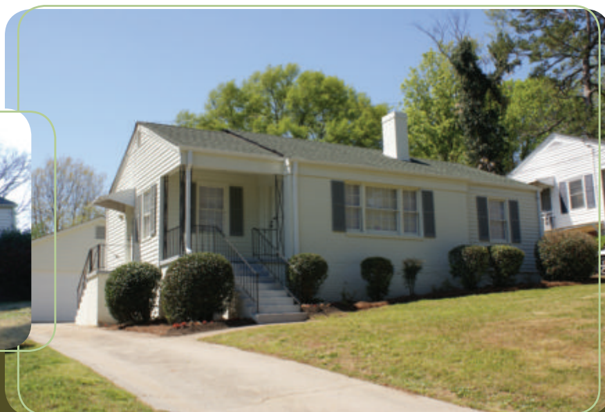
After home rehabilitation
